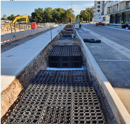
Often tree beds are incorporated into streetscape systems that include an underlying stormwater system which connects several boxes (as shown to the left). This is also coupled with pervious concrete to increase the ability of the system to intercept and capture stormwater.
